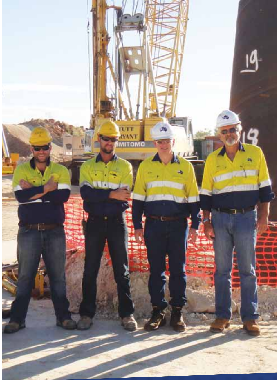
Peter Thomas visits the WPCS and Macmahon team at Coonarie Creek where bridge construction is underway.
